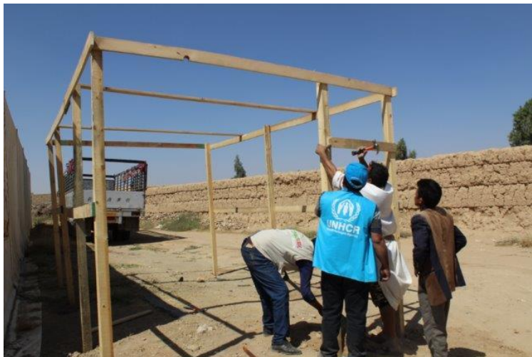
Training program on the setup and installation of the new Enhanced Emergency Shelter Kit (EESK) in Sa'adah, Yemen. © UNHCR/ Abdullah Thawabah
