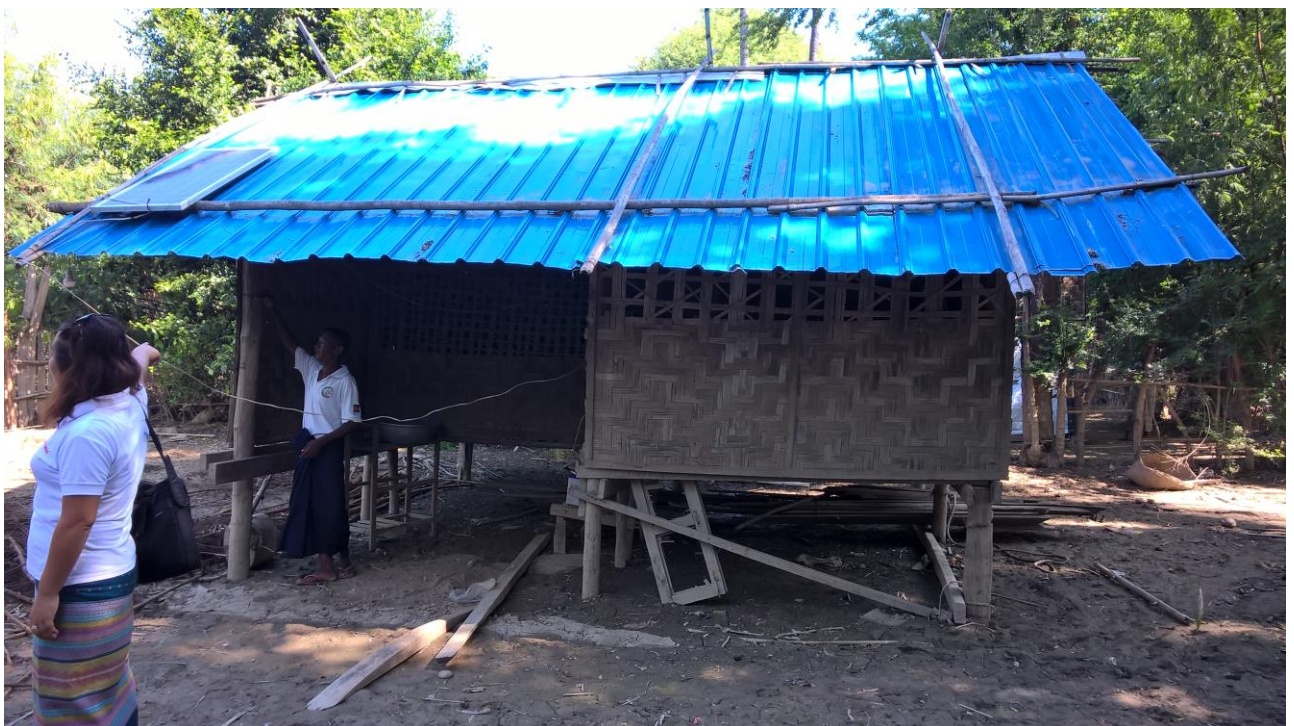
Reconstructed house in Kyun Ka Lay village, Pakokku Township. House not elevated sufficiently. Photo taken by Shelter Cluster.
