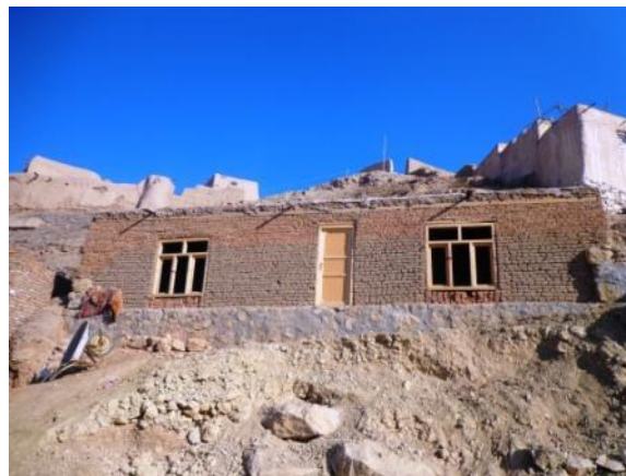
Mountainside shelter in Pul I Khumri, Baghlan Province (Photo: SHA)
