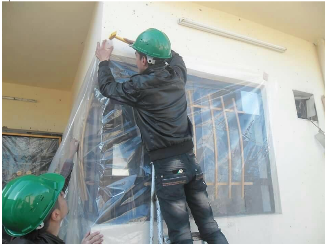
Local workers in East Mosul undertake emergency shelter repairs on homes.
