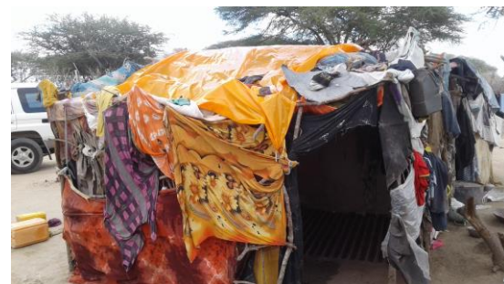
Typical makeshift 'Buul' with cloth roof and walls
