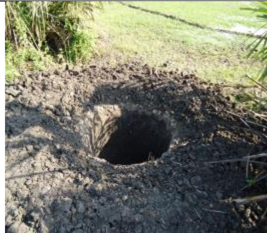
Figure 5 local latrine construction
