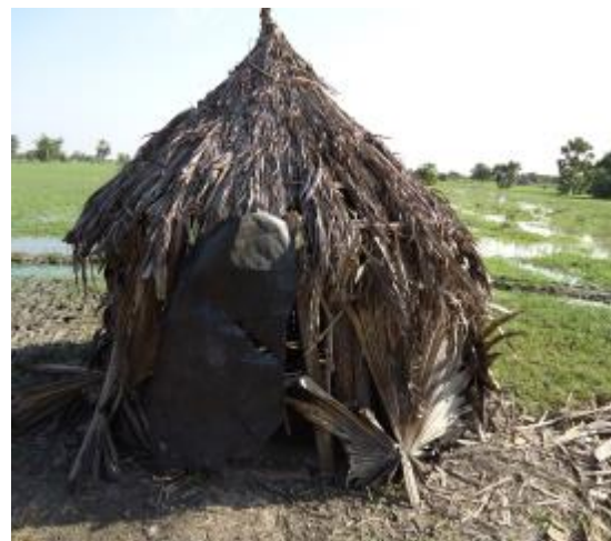
Figure 6 Complete local latrine
