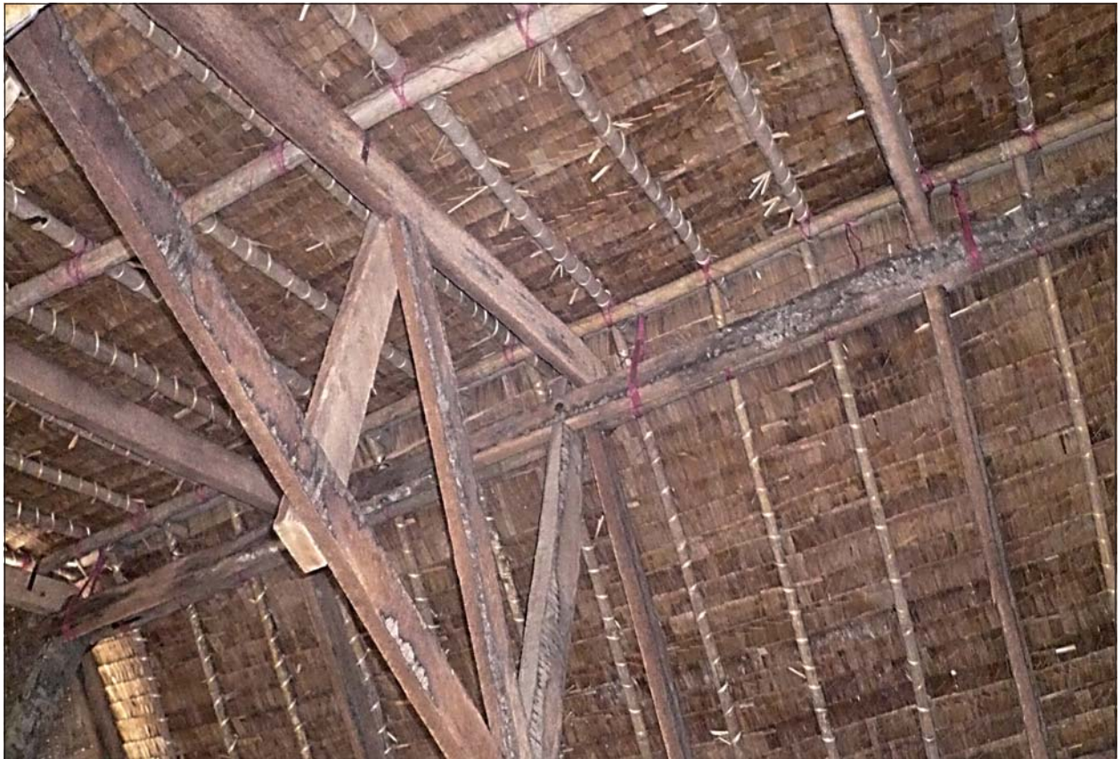
"Dani" roof viewed from inside ▲
