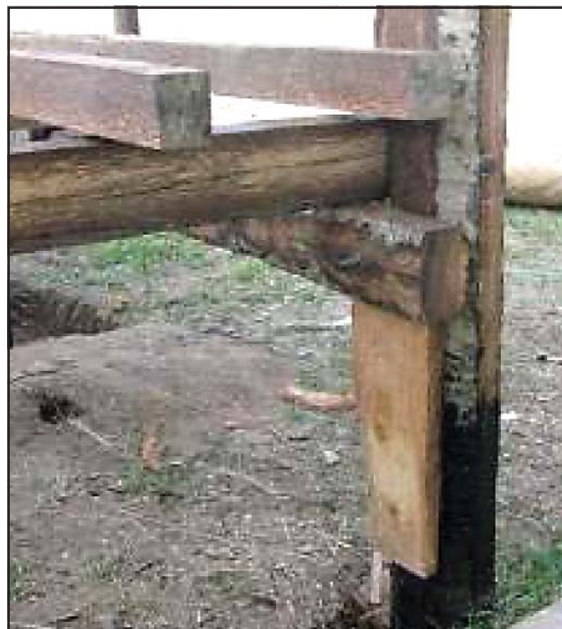
Cross joist and long joist mounted on post with nuts & bolts and cleat ▲
