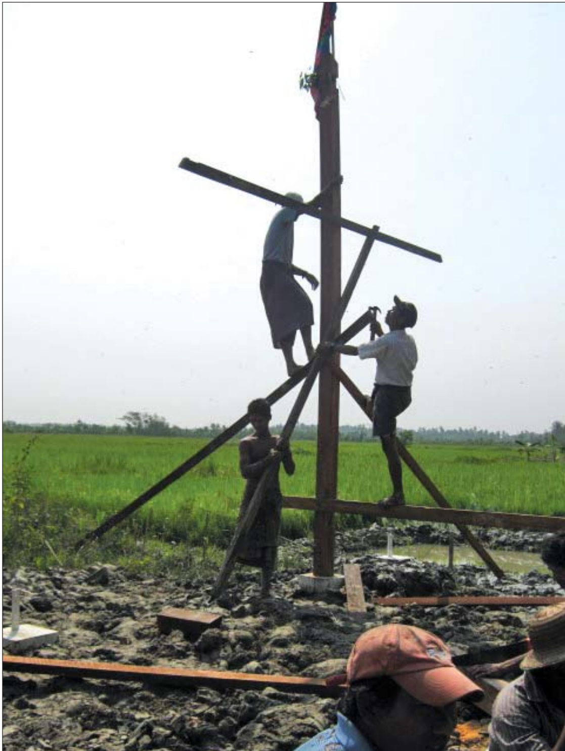
Posts held in position with temporary supports ▲
