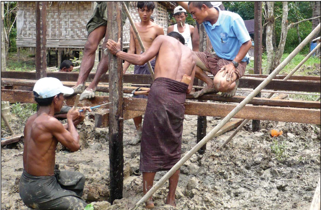
Fixing floor joists ▲
