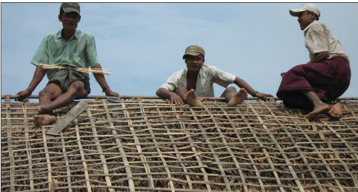
"Dani" covered roof ▲
