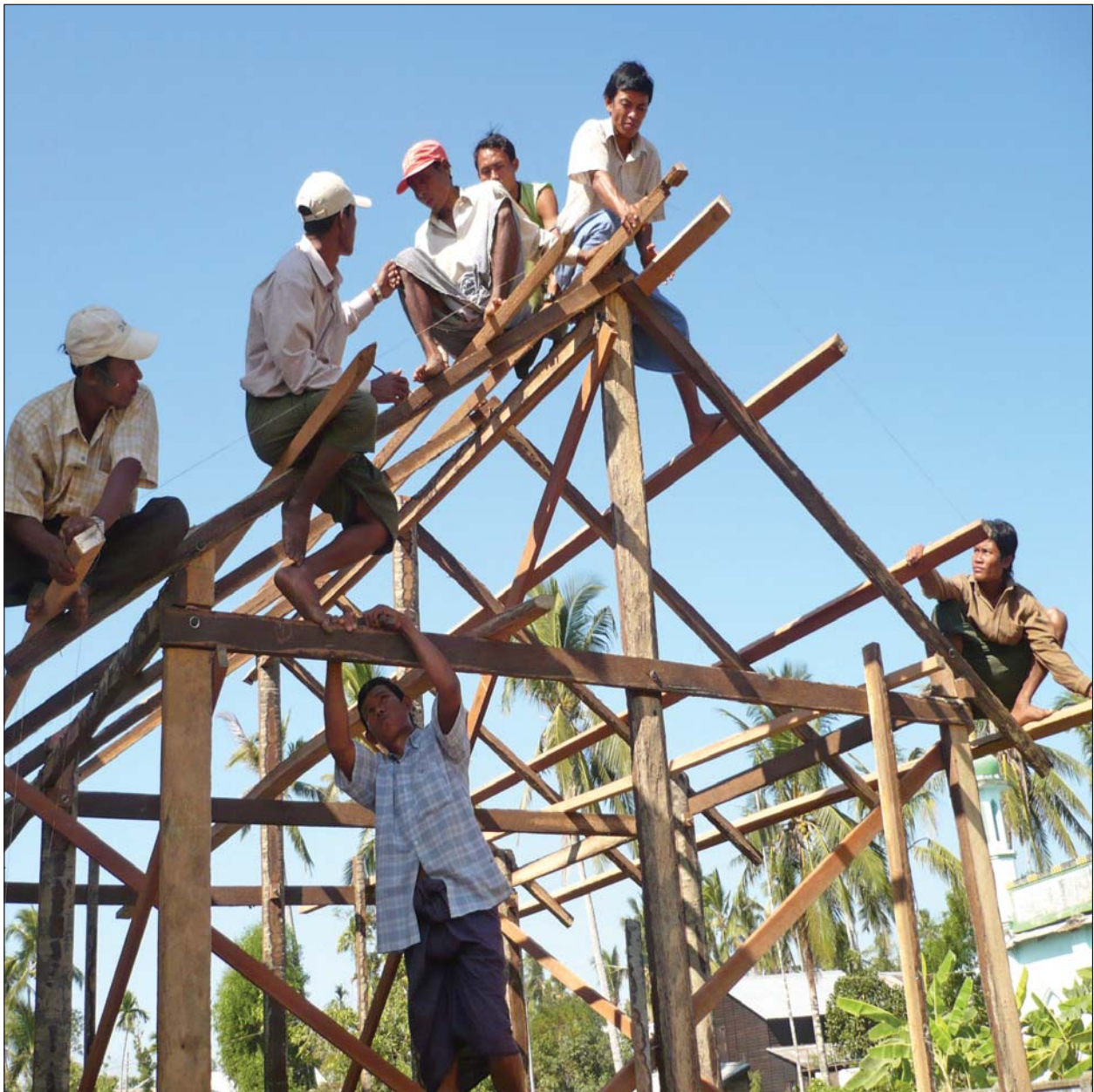
Pair of rafters being erected ▲
