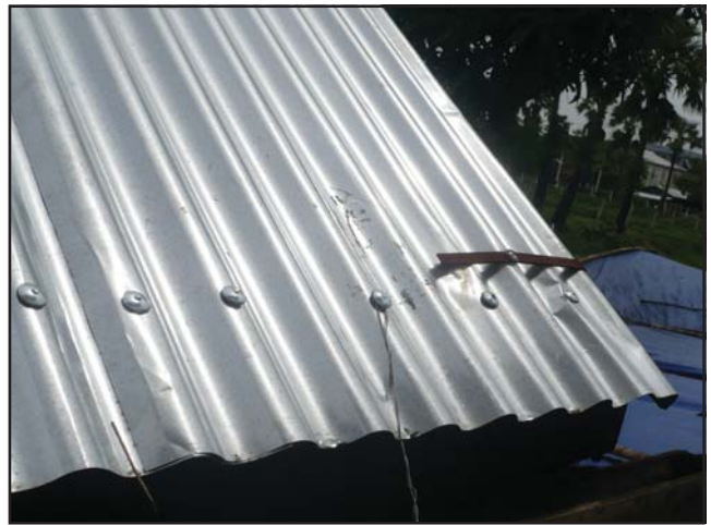
Roof with CGI-sheets ➤
