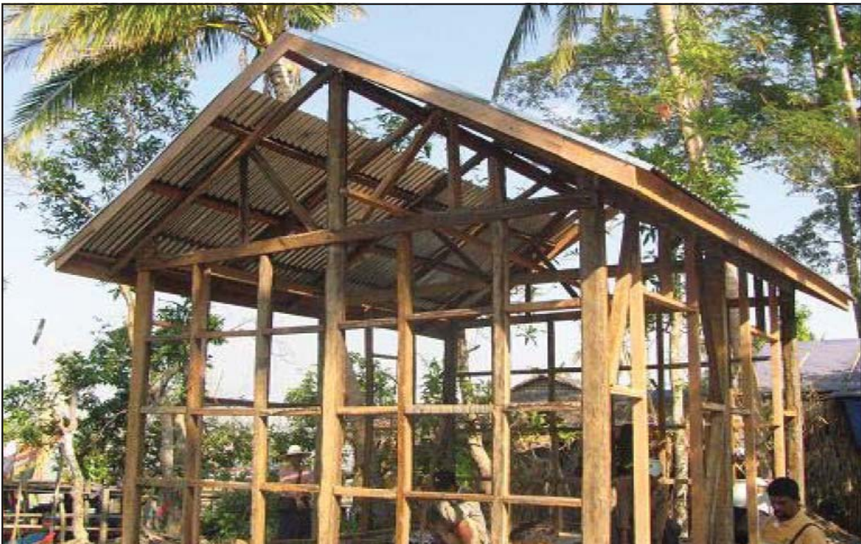
Framework for wall cladding ▲
