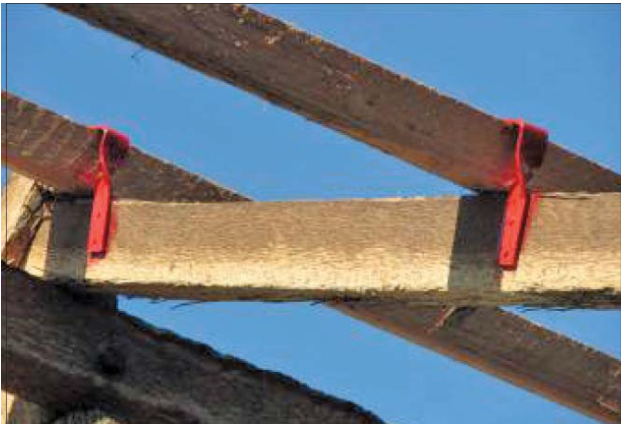
Steel straps to anchor runners to rafters ▲
