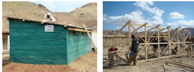
ARC Shelter Project Plan vs Completed status (153 completed)
