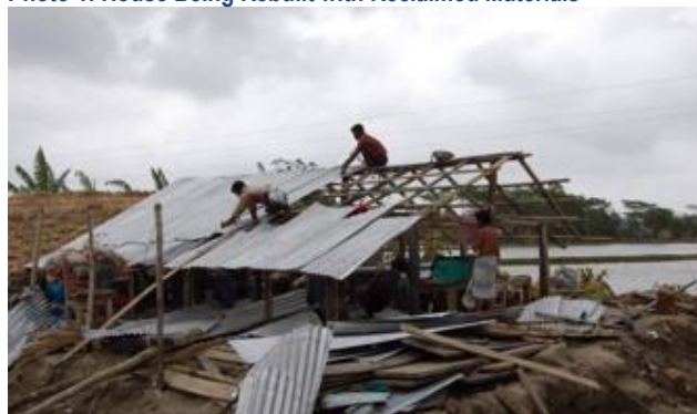
Photo 1: House Being Rebuilt with Reclaimed Materials
