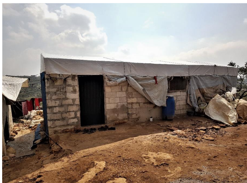
Figure 1: Self Built Shelter in IDP site in NW Syria. Credit: IhsanRD
