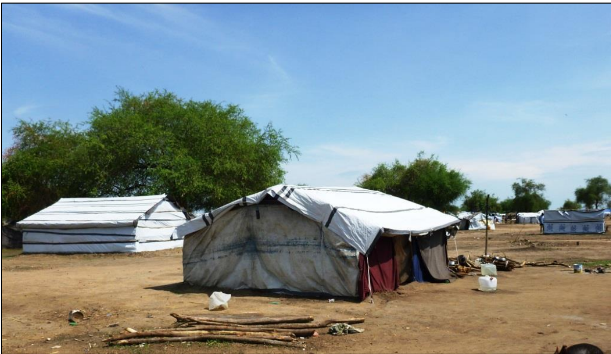
Typical shelters in Mingkaman IDP area: one using a variety of covering fabrics, including old and new plastic sheets, likely carried from home and received in distributions. The other appearing freshly constructed using materials distributed humanitarians.
