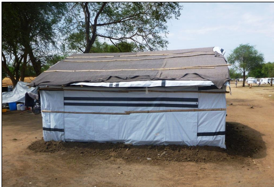
The assessment team observed that many households were using several blankets to cover their shelters to both cool the inside of the shelter and to protect the plastic sheet against sun. It appears that these blankets were not recorded in the table about NFI possession as they were not being used for the intended purpose of sleeping.
