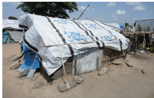
Mud and stones are used for better stability during rain.
