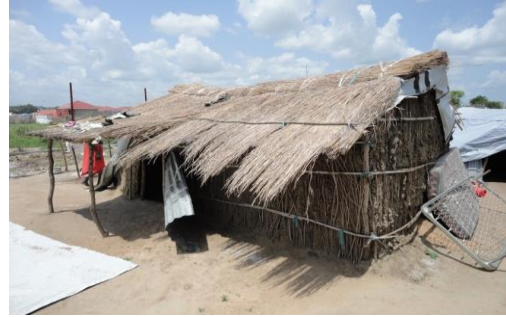
One of the shelters was improved with mud walls.
