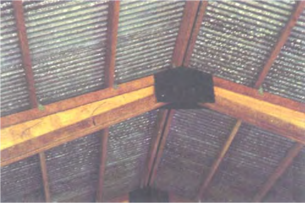
Photo 25: I-beam with plywood webbing
