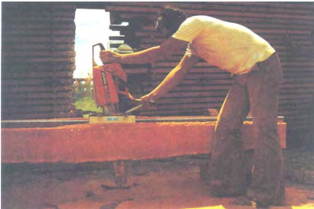
Photo 30: Chain-sawing of palm stems with guide bar
