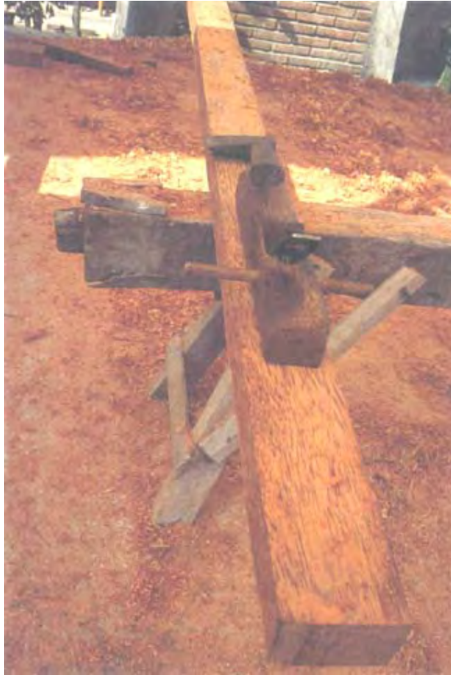
Photo 3: Handplaning of coconut beam for low-cost house construction
