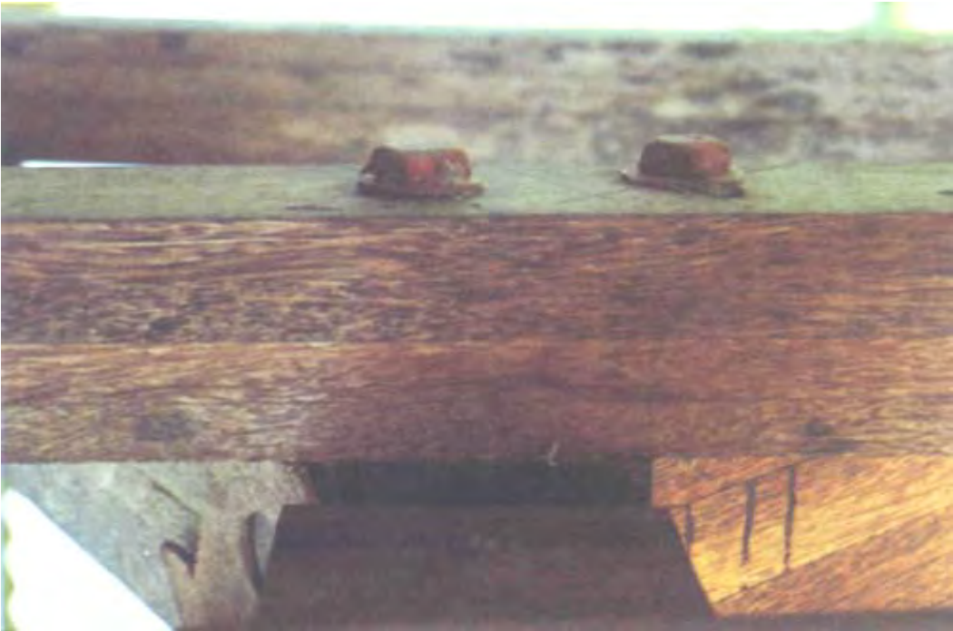
Photo 23: Laminated and bolted coconut boards
