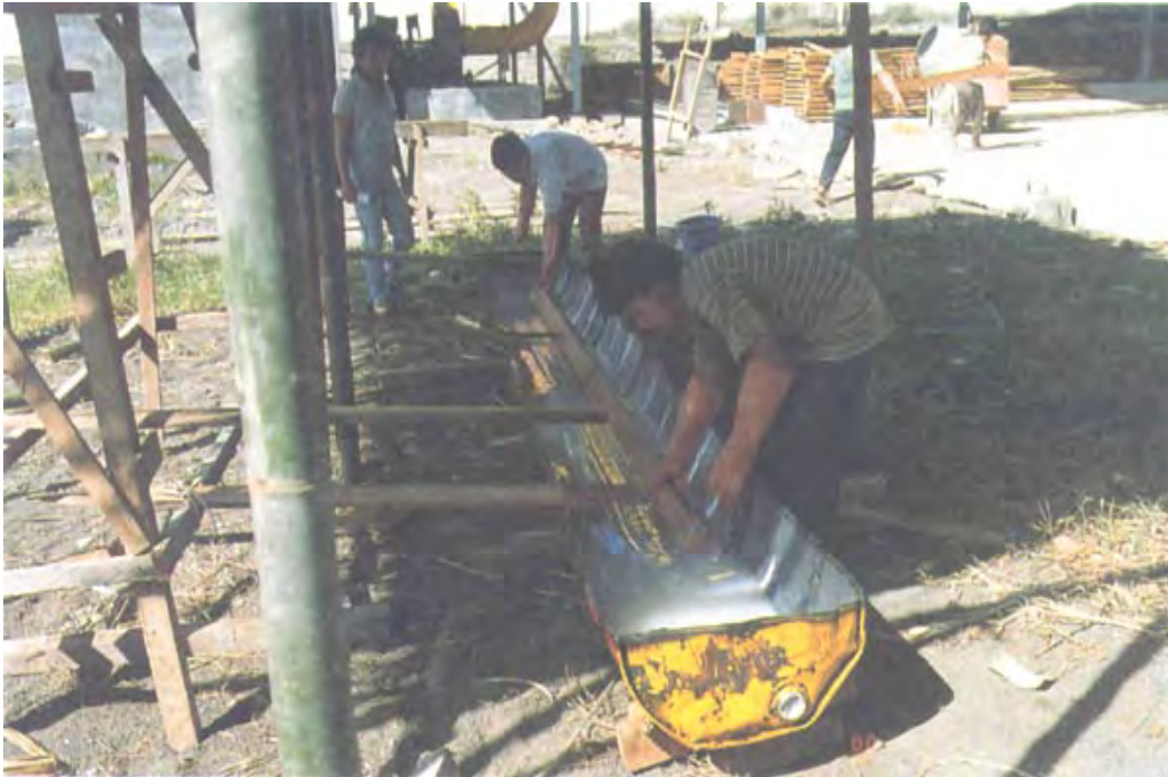
Photo 42: Dip treatment of coconut boards
