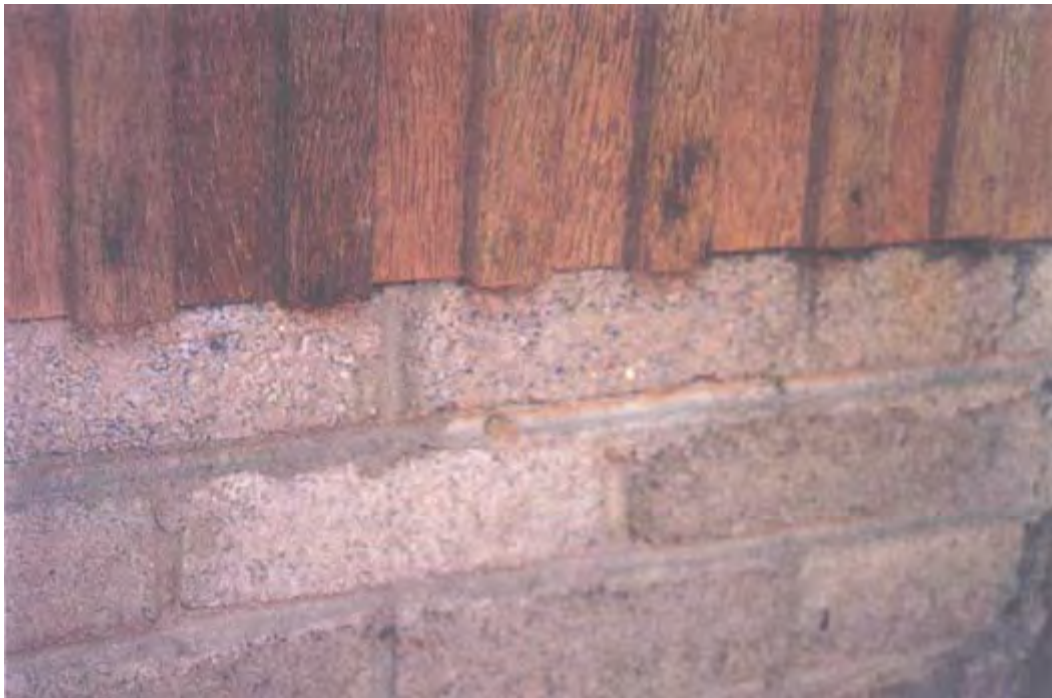
Photo 7: Detail of wall with bricks made of coconut sawdust and wall-panelling
