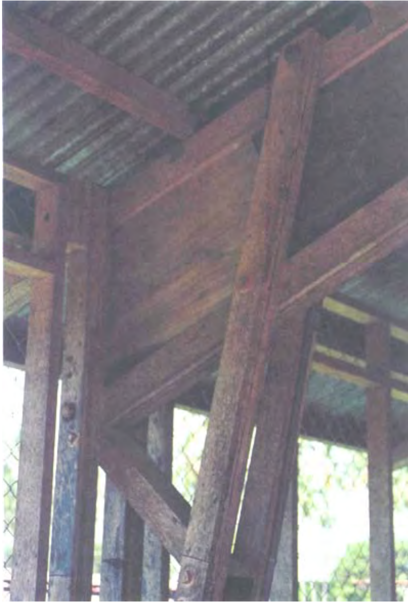
Photo 26: Laminated and bolted roof construction
