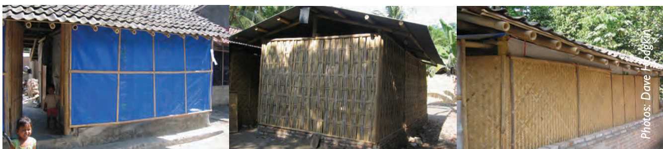
Grants were provided to build transitional shelters. Many different and innovative designs were built.
