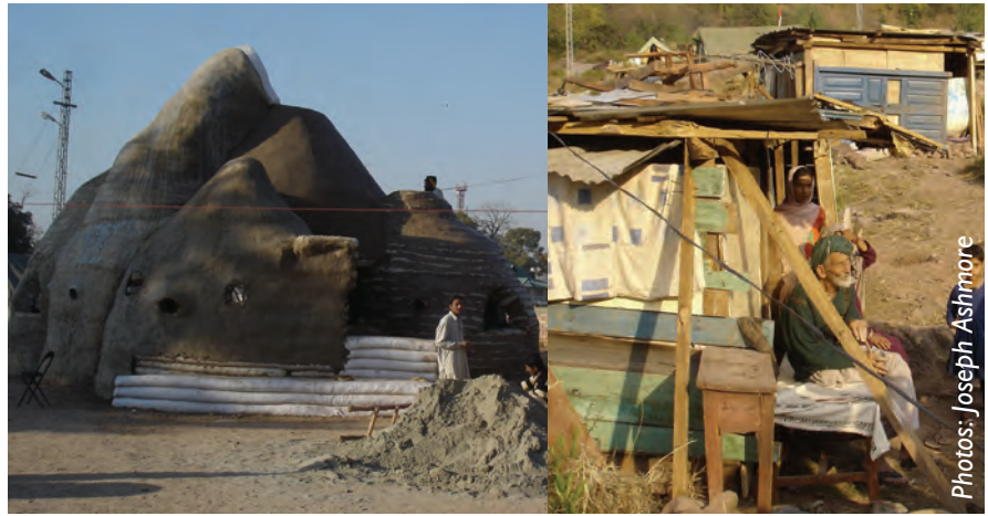
Left: Design for a timber-free domed shelter proposed as a response to an earthquake in 2005. Affectees were not involved in the design and it was not used on any scale.
