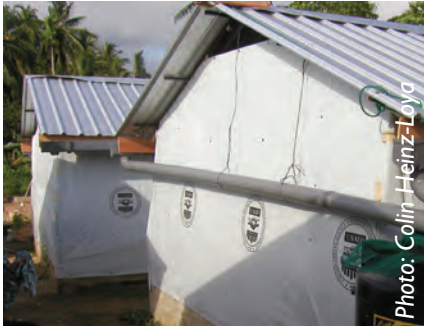
Shelters built with tanks for rainwater harvesting
