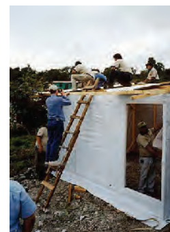
Covering the roof with corrugated iron
