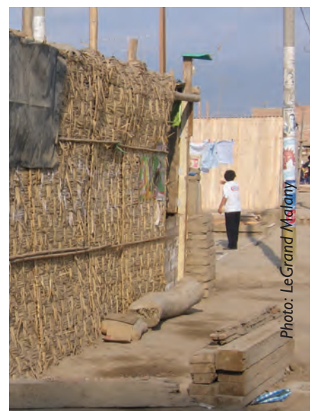
One of the project's shelters (background) and a shelter walled with reed mats (foreground)
