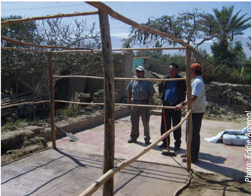
Round poles, not sawn timber, were used
