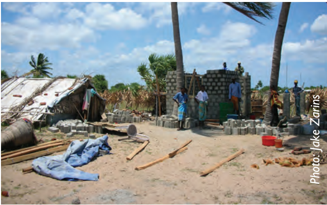
Core shelter under construction
