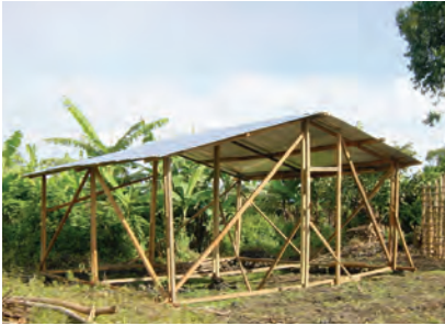
Structural skeleton of a house, showing cross-bracing
