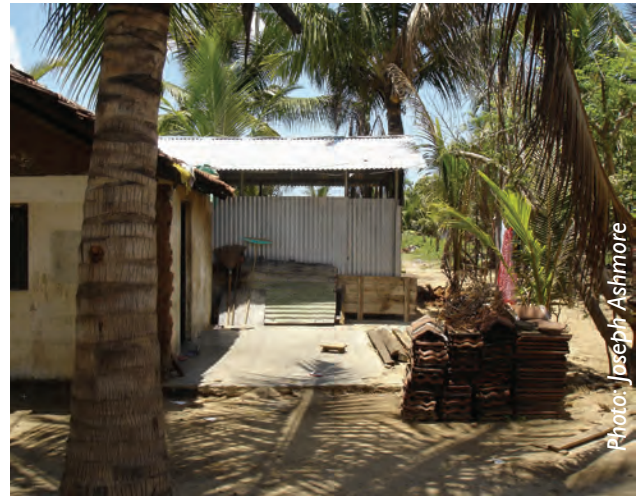
In some cases, small groups of transitional shelters were built on small plots of land that were negotiated on a temporary basis.
