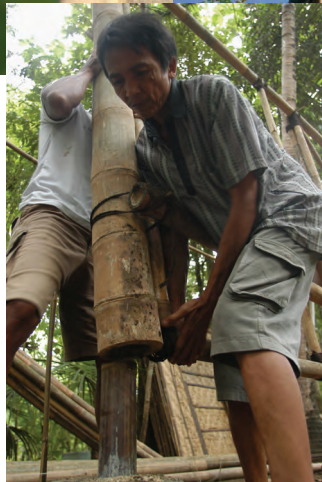
Connecting a vertical post to the foundation
