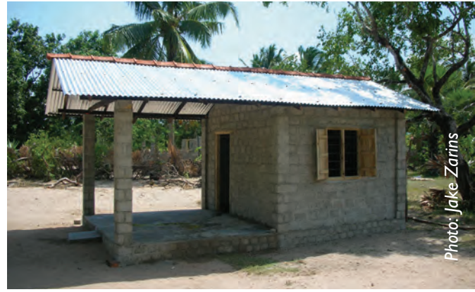
Completed core shelter
