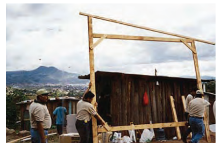
Shelter assembly using prefabricated walls
