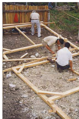
Prefabricating walls
