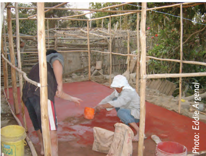
Making the concrete floor slab
