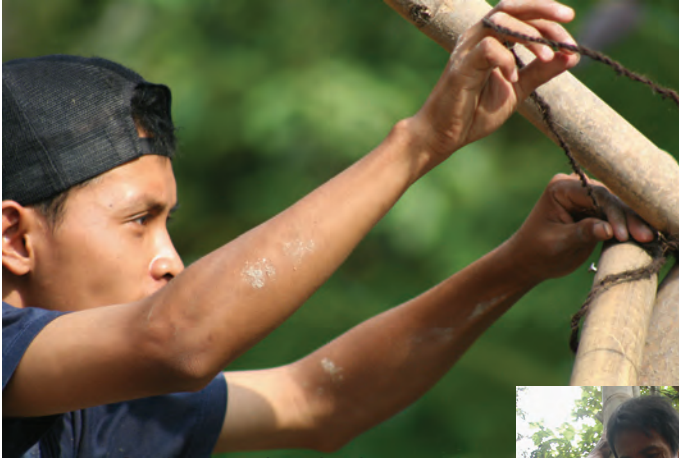
Bamboo being bound with string
