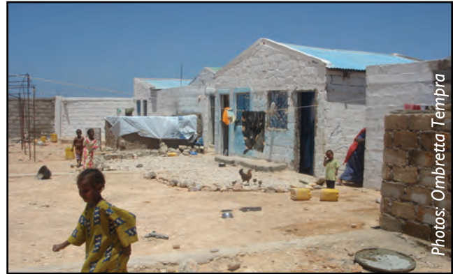
Sites and services: the project focused on negotiating land and providing access, secure compound walls, water and sanitation.
