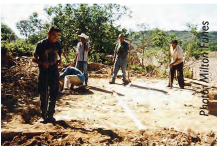
Marking out the site for a shelter
