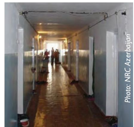
Corridors before and after upgrade
