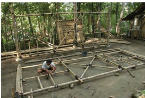
Prefabrication of a wall panel
