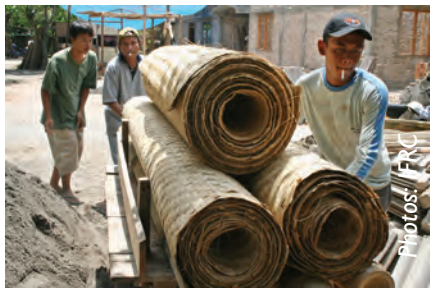
Transporting bamboo mats to a construction site
