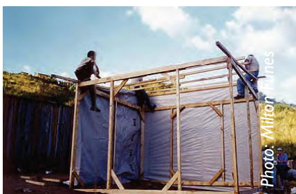
Covering the frame
