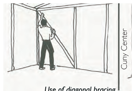
Use of diagonal bracing
