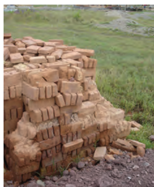
Obtaining good quality building materials remained problematic. These bricks decayed rapidly in the rain.
