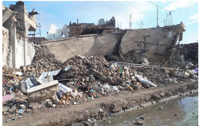
Category 4: completely destroyed/rehabilitation not feasible
