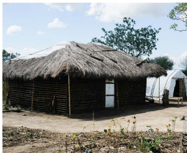
Emergency Shelter and Semi-Permanent Shelter (self-built) as part of the upgrade strategy within the same household, Ntokota Relocation Site, Metuge, Cabo Delgado.
