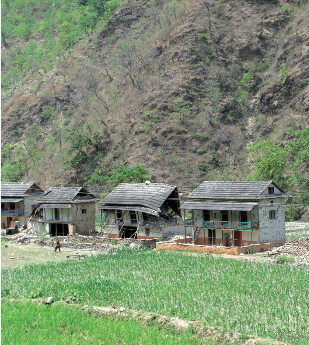
Nepal, after the 2015 earthquake
