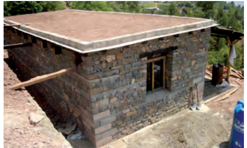
Pakistan, after the 2005 earthquake: damaged house and newly rebuilt house with improved stone masonry
