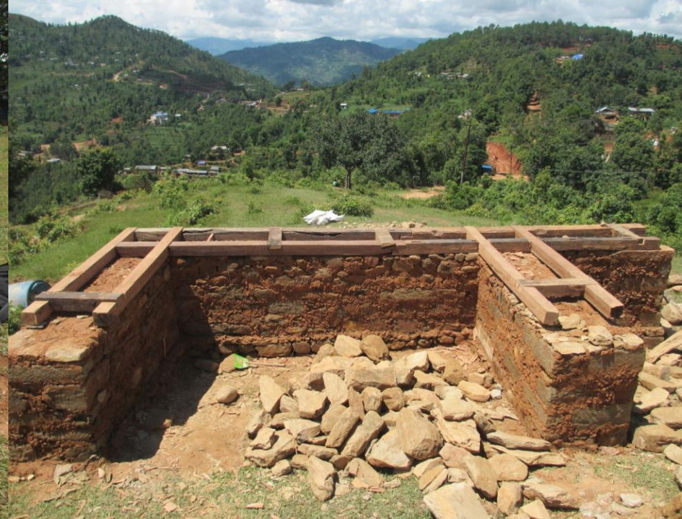
5. Completion of first layer of wooden seismic band.
