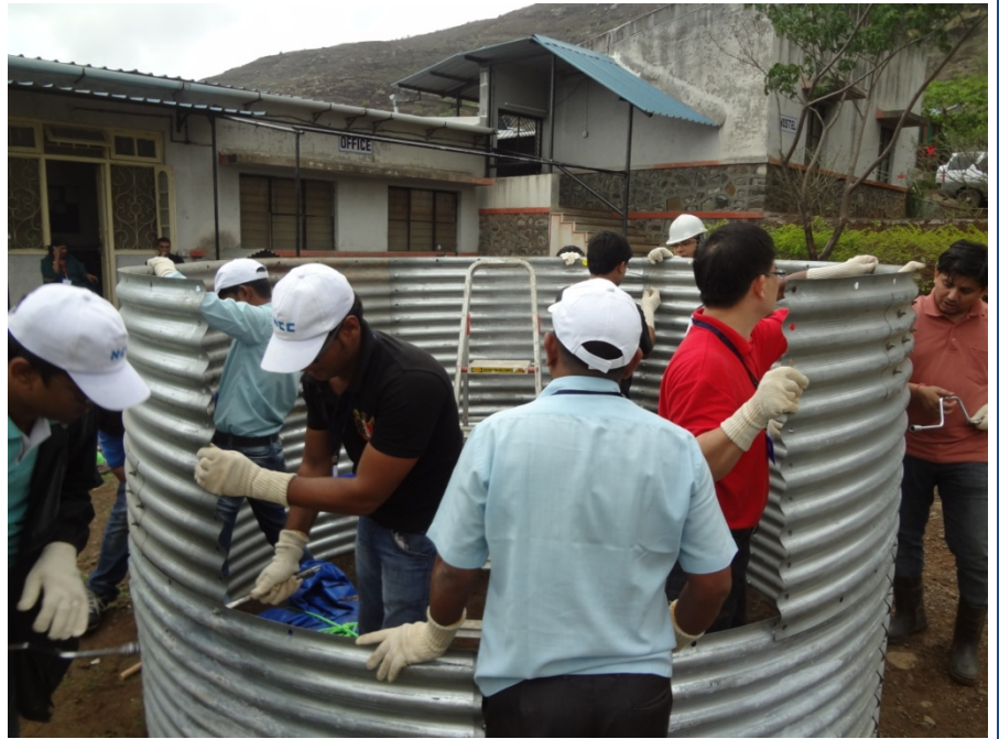
Engineers from the different DRN-India companies – including the first ever female participant – installing a T11 Water tank (above) and building emergency latrines (below).
