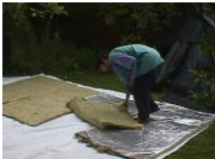
constructing doors with mineral fibre duct wrap and UNHCR sheeting
