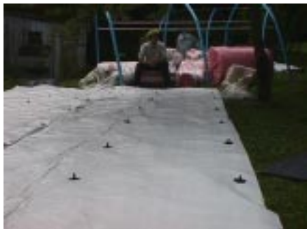
Monarflex universal sheeting with poly toggles/ snap-fitted to eyelets
