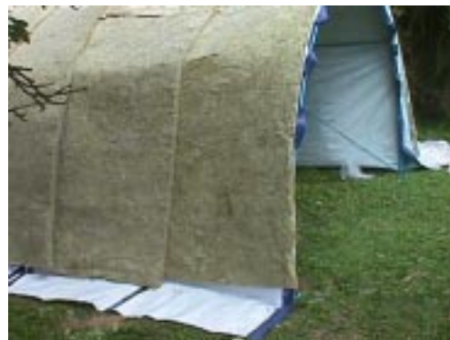
four lengths of mineral fibre cover the roof with overlap joints to prevent cold bridging
