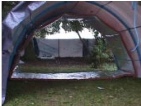
glass fibre duct wrap forming roof and floor insulation in one section
