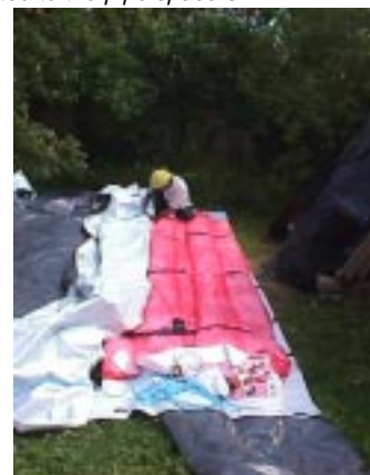
top sheet toggles are snap fitted to the pipe spacers
