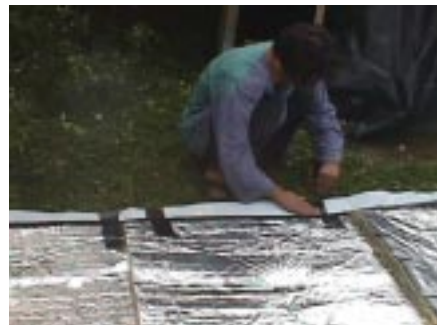
four lengths of mineral fibre cover the roof with overlap joints to prevent cold bridging
