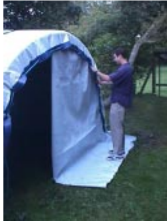
25mm duct wrap is light enough to construct doors
