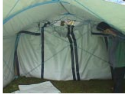
mineral fibre is too heavy to be used as door insulation as it pulls itself from the structure
