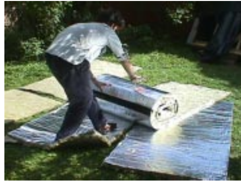
insulation comes in 1x4 metre rolls
