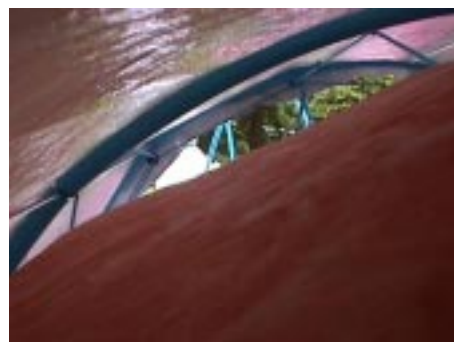
ventilated gap between roof sheet and insulation
