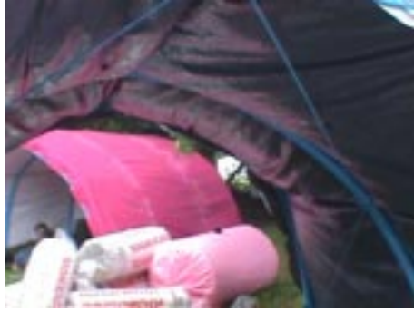
the erected shelter showing insulation sagging into the living space
