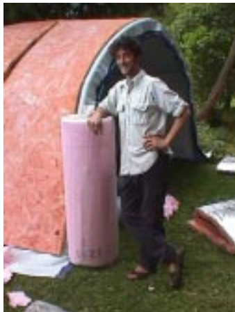
glass fibre duct wrap is thrown over the first roof sheet. The packed roll is shown at the fore front
