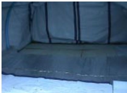
experiments with mineral fibre products for flooring insulation
