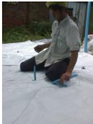
20mm pipe spacers push fit over the poly toggles
