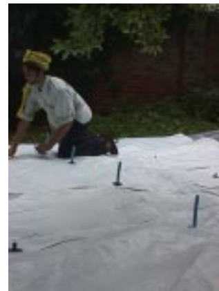
20mm pipe spacers push fit over the poly toggles
