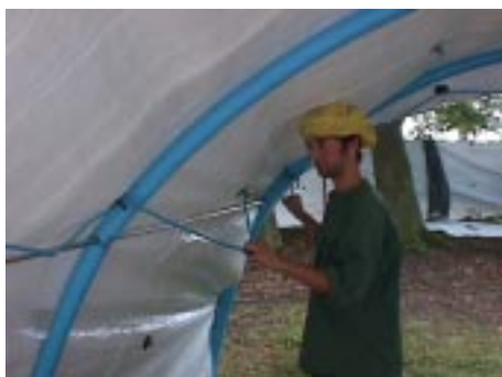
polypropylene rope is attached to the roof sheet using poly-toggles
