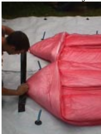
insulation is taped to sheet to minimise differential movement during construction/
