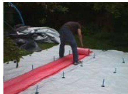
resin free glass fibre is rolled between the spacers
