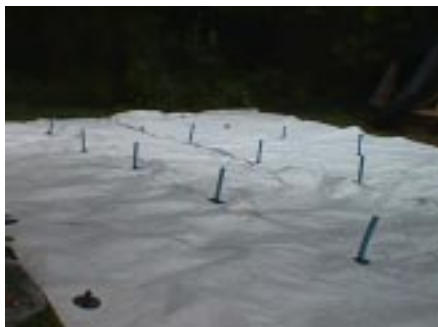
Monarflex universal sheeting with poly toggles/ snap-fitted to eyelets
