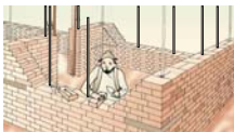
Lay the walls straight in plumb and at right angle. Make steps as shown in picture and then fill the middle part
