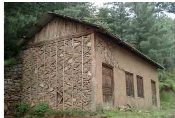
One of the few examples of pre earthquake Dhajji construction, used for research purposes in the development of standards for reconstruction,
