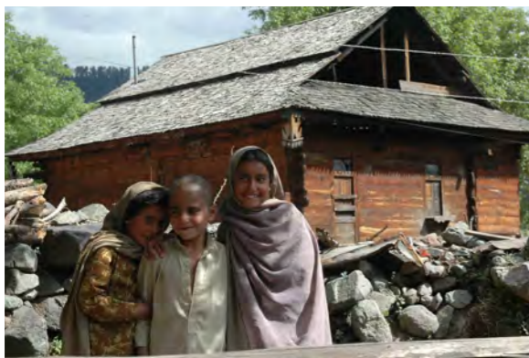
Traditional Leepa house with shingle roof and open gable, 905 new houses were constructed in the same way in this valley.
