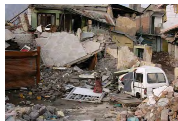
The collapse of reinforced concrete and masonry buildings in small towns was as extensive as the damage to weak traditional construction,
