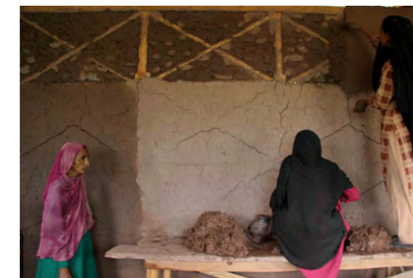
Traditionally women carried out plastering and finishing of houses. The regeneration of local technologies was matched with reviving these skills.
