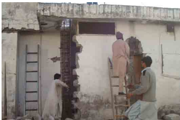
Repair and retrofitting training at damaged house, Muzaffarabad. High building costs meant retrofitting was usually economical if damage was not severe.
