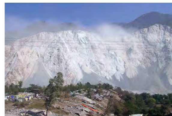
Chela Bandi village, north of Muzaffarabad, land lost in sliding, severe damage to village, all residents left homeless.
