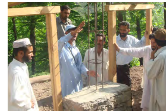
UN-HABITAT Assistance and Inspection engineer advising mason, houseowner while construction is underway, to clarify standards required for certification
