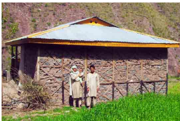
The approval of safer and improved local technologies by ERRA ensured reconstruction was affordable by low income families, including use of salvage.
