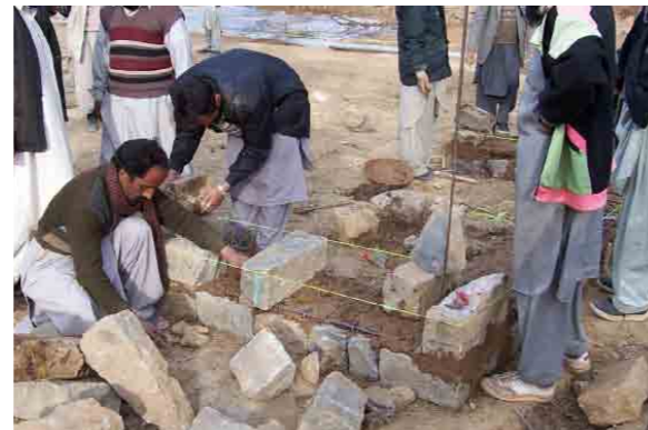
Training at HRC: through stones in masonry, reviving old knowledge the loss of which had contributed to the poor performance of buildings in the earthquake.
