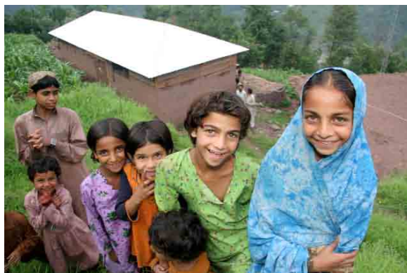
Very low income families in remote areas managed to construct basic ERRA approved houses, and can upgrade or extend in future according to resources.
