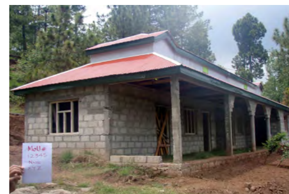
Final formal ERRA inspection at lintel level not roof level. Sample roof level completion survey carried out showing over 80% full completion end 2009.
