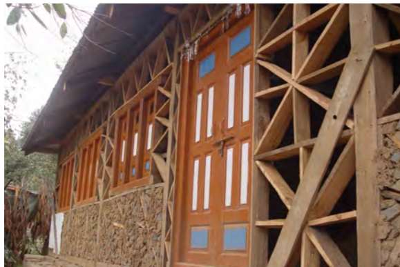
One of the 128, 500 Dhajji houses timber frame infilled with stone and mud, all walling materials recycled from salvage. Sustainable technique using local skills,
