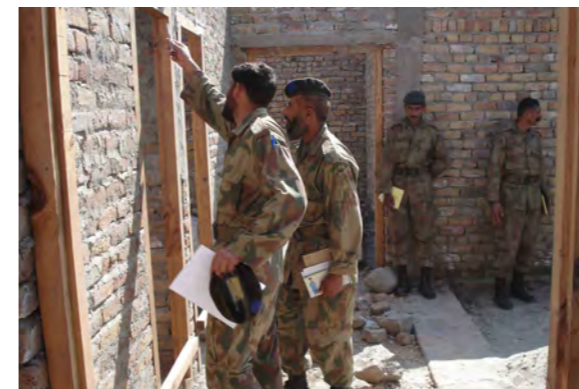
Army Engineering Assistance and Inspection (AI) teams in training to ensure consistency in inspection criteria and application of ERRA standards.
