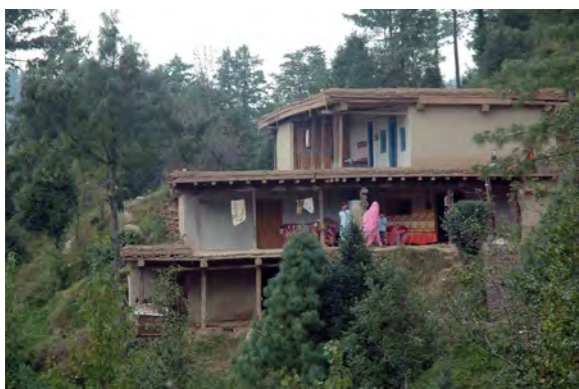
Pre-earthquake housing in the affected area unreinforced masonry, large extended family dwelling built on steep slopes, often multi storied.
