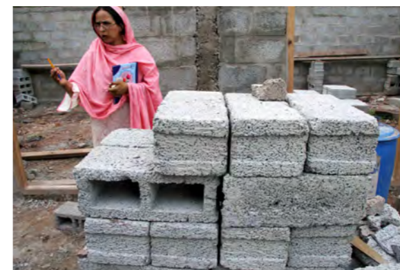
Women headed households faced the challenge of organising materials and labour. With access to finance and technical advice they managed successfully.
