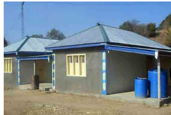
Rainwater harvesting on newly reconstructed house, optimizing the potential of new cgi roofs. Rainwater storage tank and first flush tank to the right of picture.
