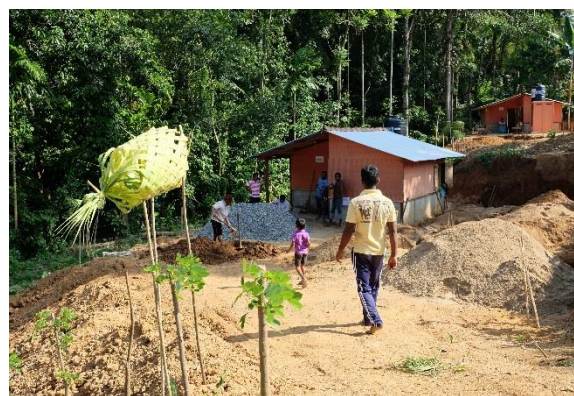
Construction under way at TS site – A. Lind © IOM, 2016
