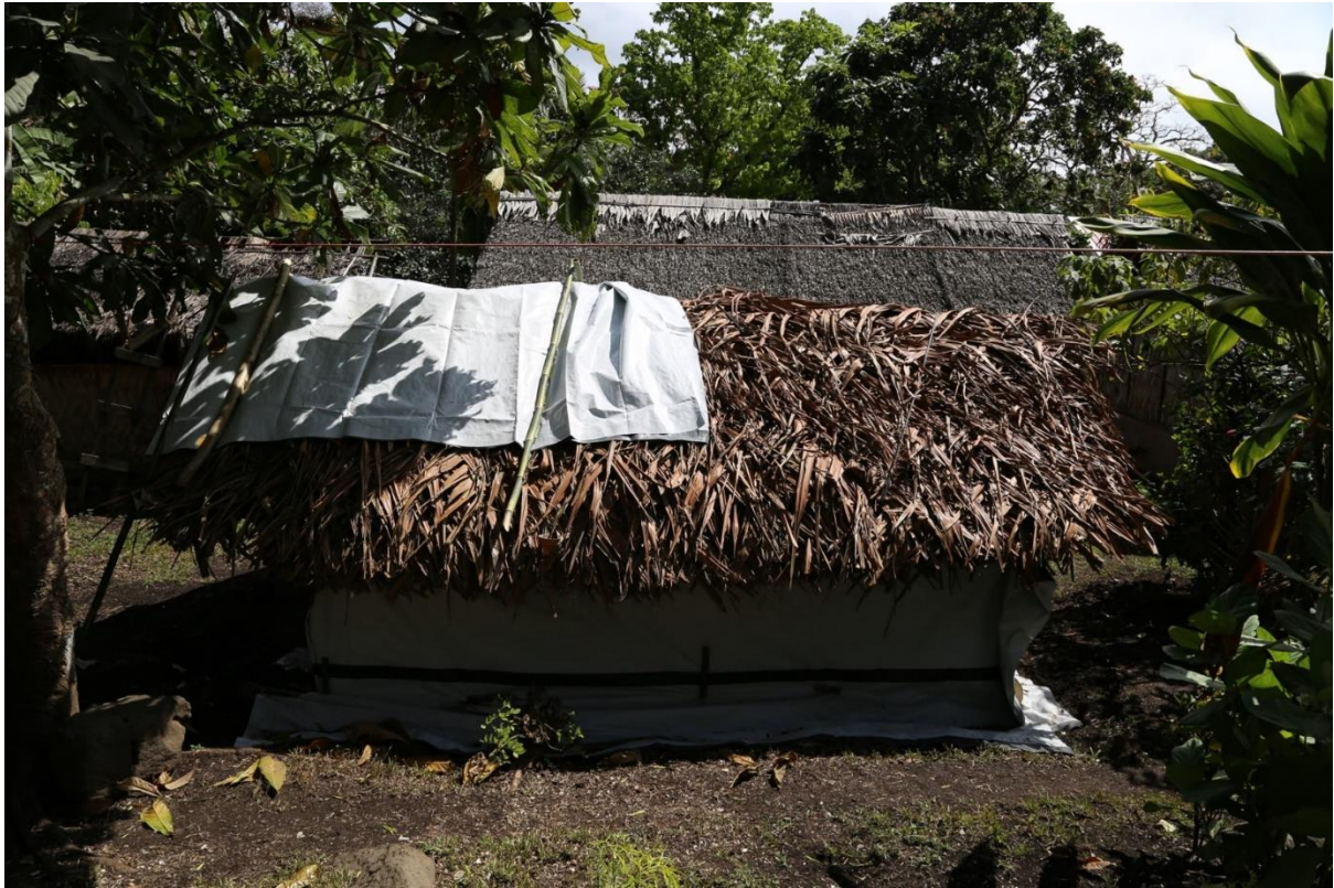
Shelters are starting to be upgraded using traditional materials from the bush
