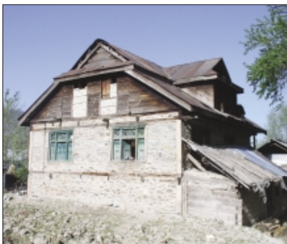
Two-sided CGI roof on timber and random rubble walls
