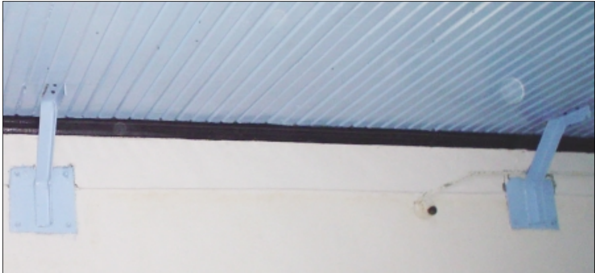
MS brackets for anchoring roof deck to wall
