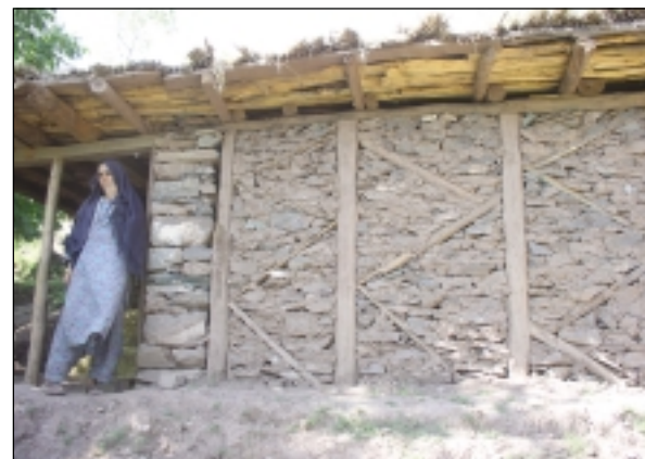
Dhajji wall in-filled with stone
