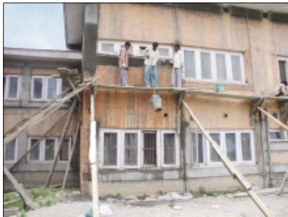
Retrofitting work in progress
