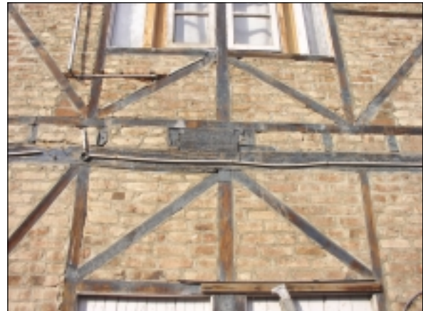
Dhajji wall with baked bricks
