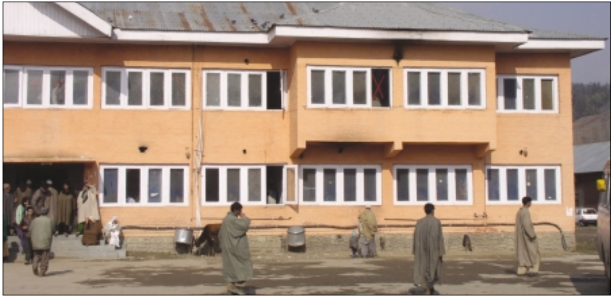
Existing building - large numbers of window openings in walls make it vulnerable
