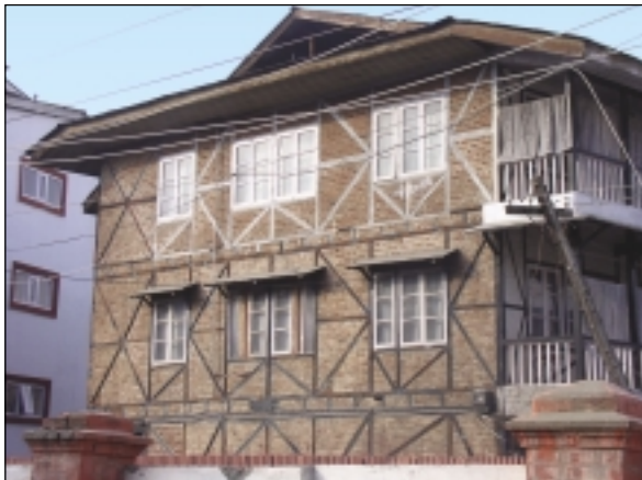
Four sided CGI roof on un-plastered Dhajji walls
