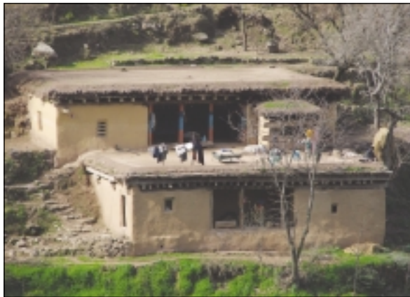
Mud roofing on timber deck placed on rubble masonry walls
