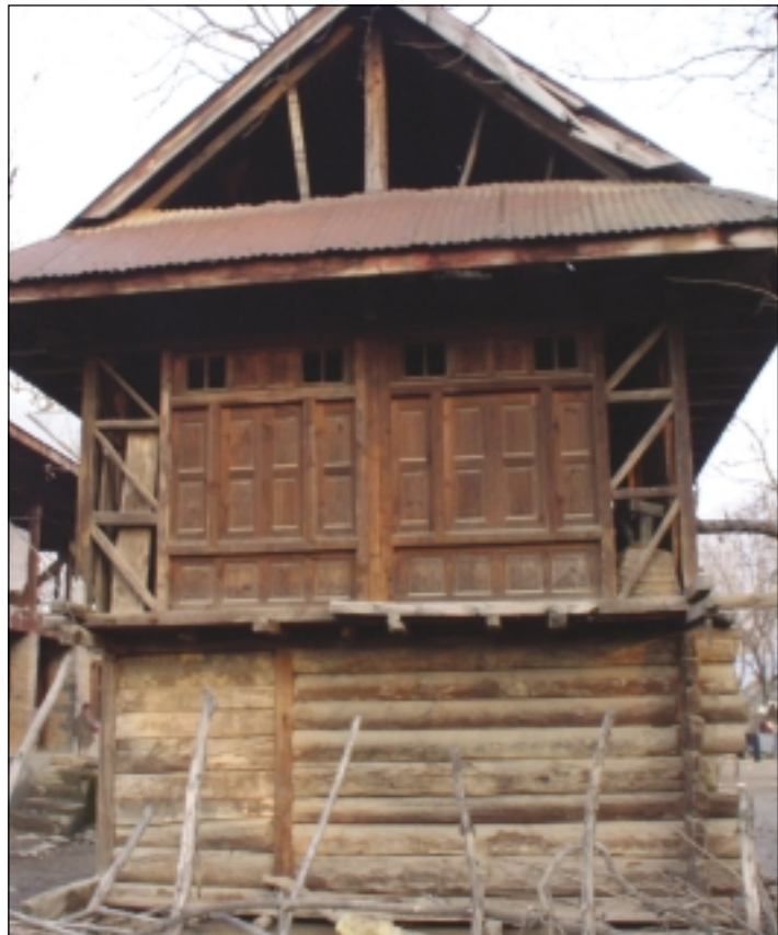
CGI roofing on timber with walls of wood planks and logs
