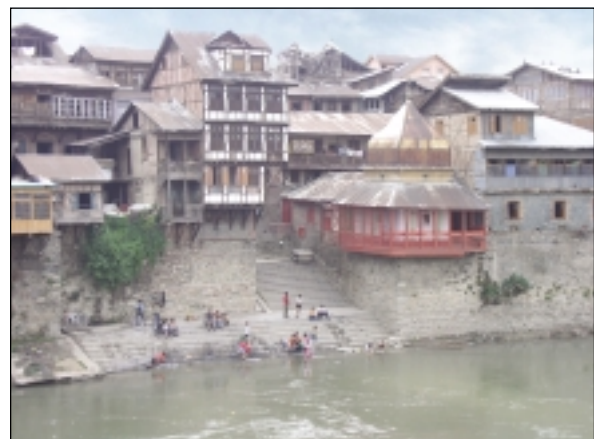
River front view
