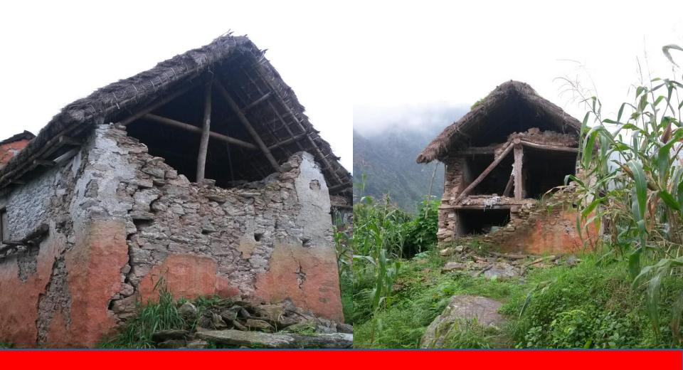
High level damage – structural collapse Less than 10% of the buildings
