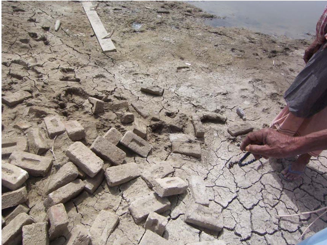
Figure 6 Salvage material from adobe houses was very limited
