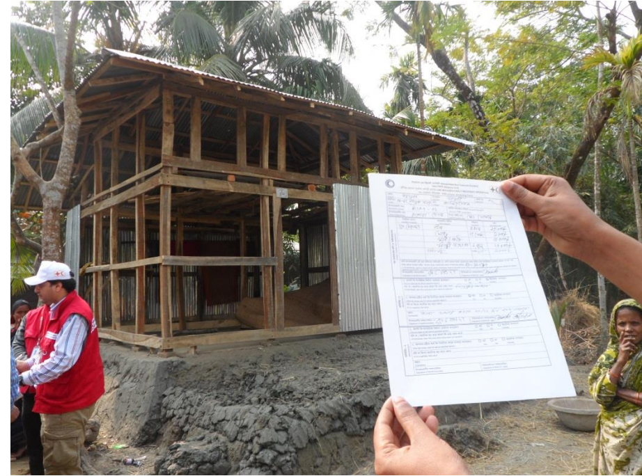
Photo B: Shelter construction is going on in Sadar upazila, Barguna District
