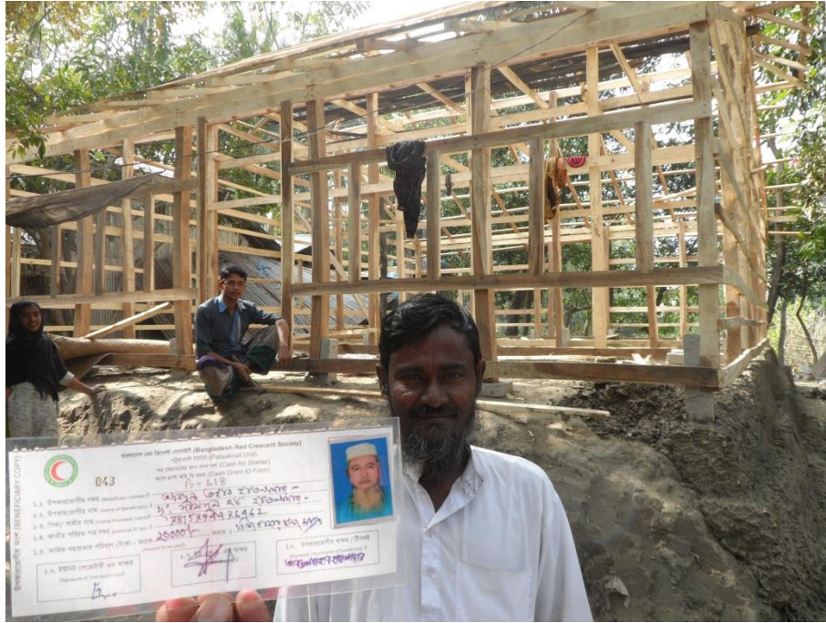
Photo A: Shelter construction is going on in Galachipa, Patuakhali District
