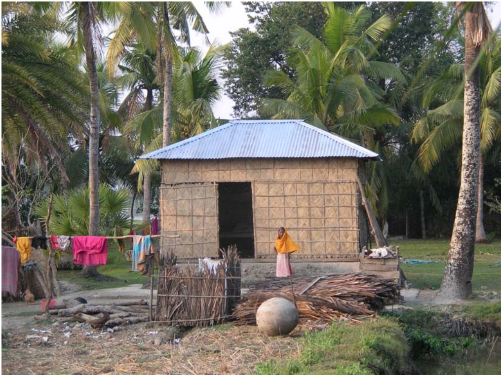
A core family shelter - UNDP phase I (all photos are by the authors unless stated otherwise)
