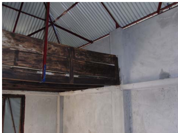
UNDP prototype family shelter showing mezzanine and steel roof
