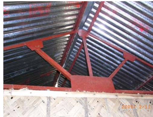
Steel roof truss - CARE
