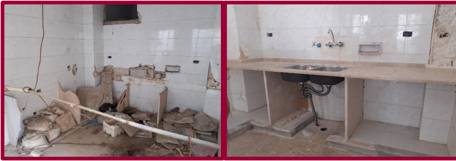
Rehabilitation of partially damaged apartments June 2021 credit: DRC Homs, Jab Aljendaly.
