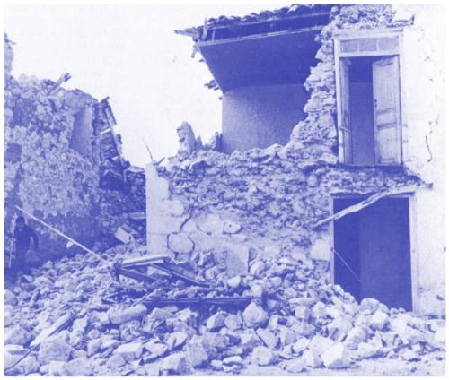
This masonry house in Corinth, Greece was badly damaged in the earthquake of March 1981. Inadequate bracking of stones, and the use of mud mortar were two reasons for the failure. Techniques can be communicated to local craftsmen on a seismic building techniques.
