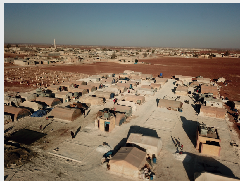
Photo Credit: Ghiras Alnahda, Site/ infrastructure improvement activities
