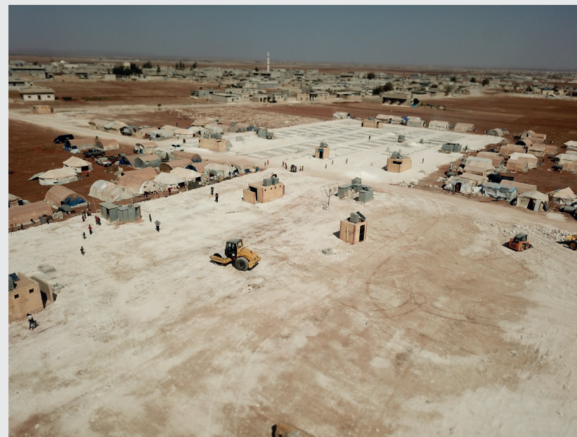
Photo Credit: Ghiras Alnahda, Site/ infrastructure improvement activities
