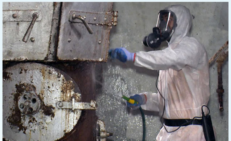
Although Fiji has relatively little asbestos, the situation identified at the Tamavua Twomey Hospital in Suva was found to be extremely high risk. PacWaste undertook remedial action at the site as soon as the problem was identified. Photo credits l-r: E.Vanderburg/SPREP; Amol Lal.
