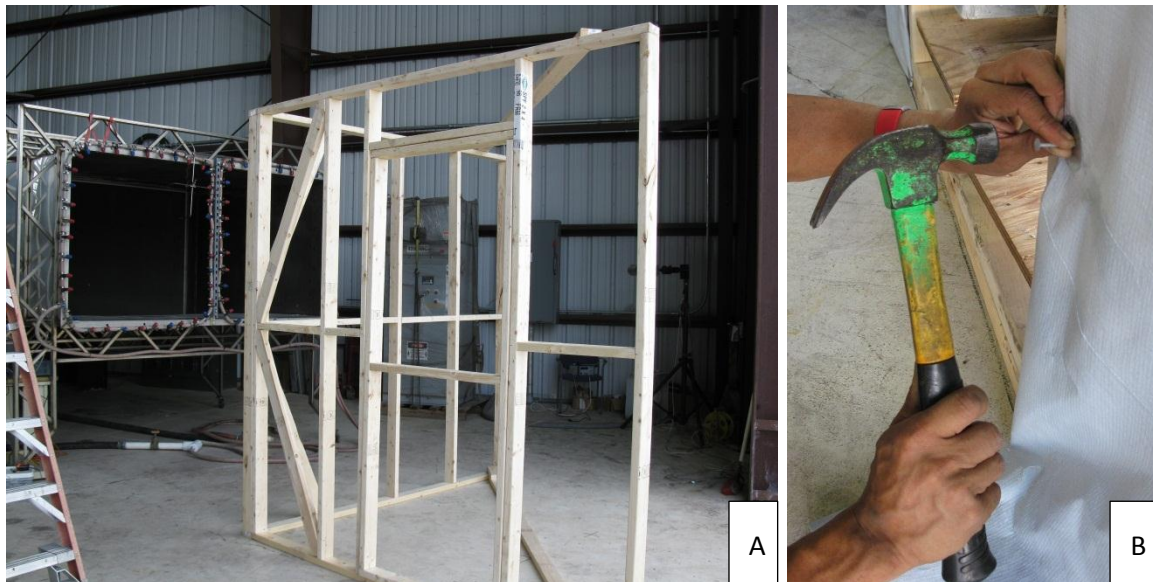
Figure 3 – (A) Shelter corner section frame and (B) sample plastic attachment
