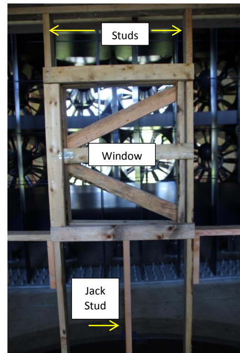
Figure 8 - Window framing
