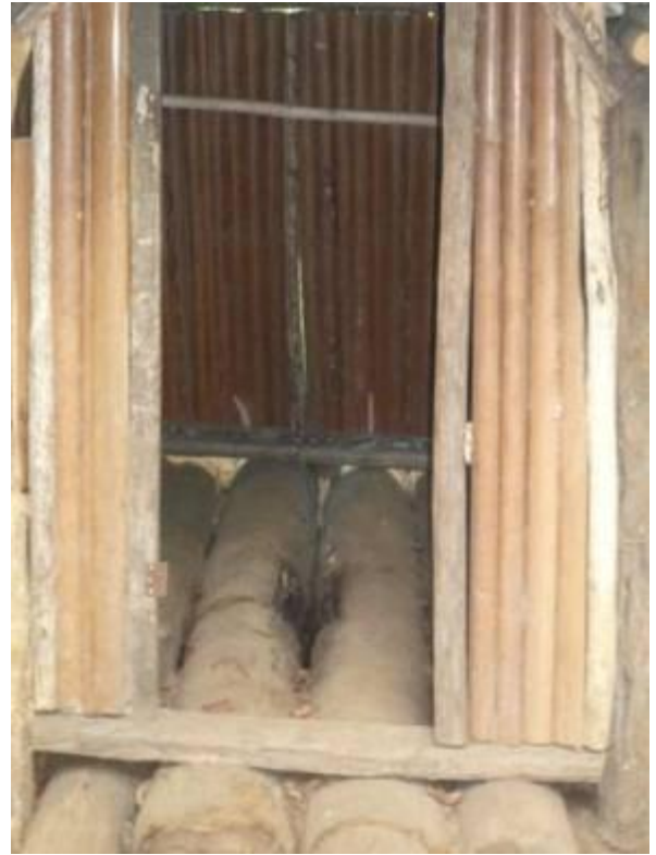
Figure 18: Locally constructed timber floor
