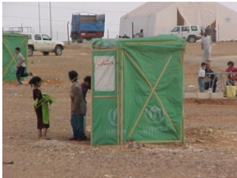
Figure 19: plastic sheeting used for latrine and washroom walls (Jordan 2003)
